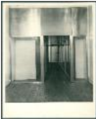
Photograph 1, 'Corridor Store Front', Photographer Unknown, 1967–68 (P09-F03-S03-0007)
